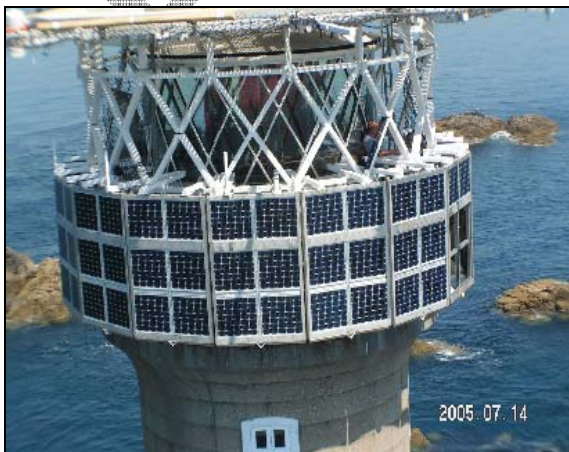
Figure 13: Longships lighthouse with solar panels to provide power to the navigational aid, main, standby and facilities battery bank. Brackets fitted for four 400W wind generators to supplement the charging regimes
