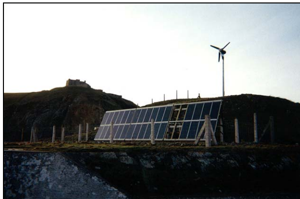
Figure 9b: Combination of a solar array and a Proven WT2500 wind turbine at Lundy South
