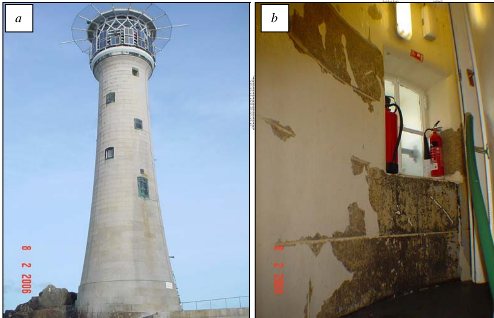
Figures 15: (a) Exterior of Hanois lighthouse and, (b) interior of the tower showing deterioration of painted surfaces
