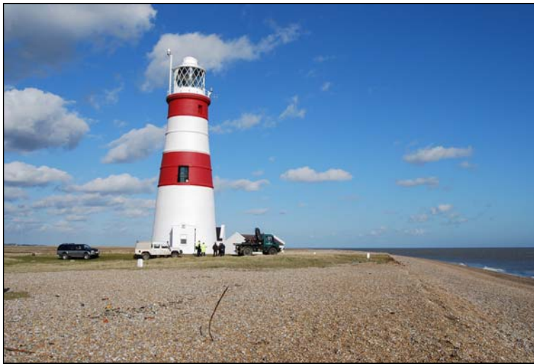
Figure 6: Orfordness Lighthouse located on a shingle spit which is undergoing significant coastal erosion that will eventually jeopardise the structural stability of the tower
